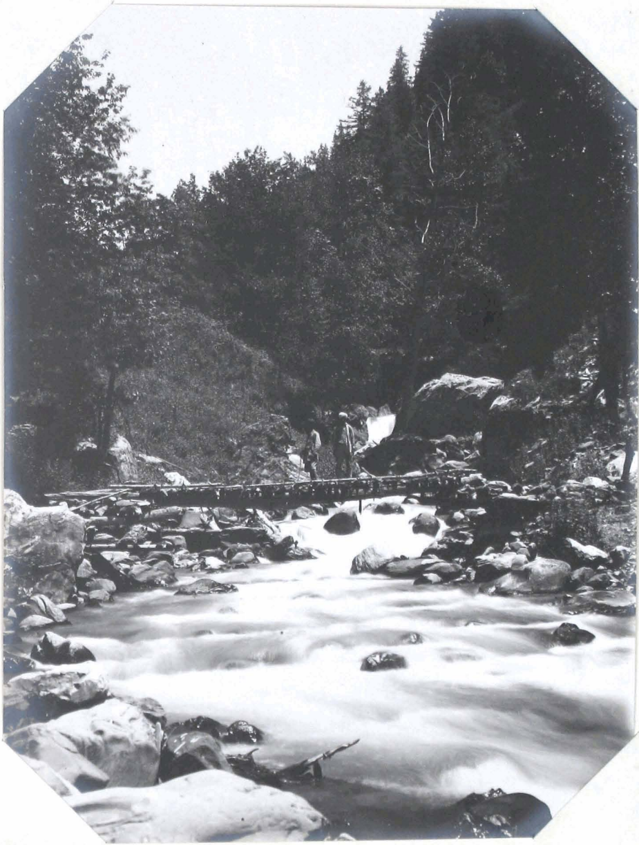
67 . LOG-BRIDGE ON THE MAREW-SINDH, WADWAN
